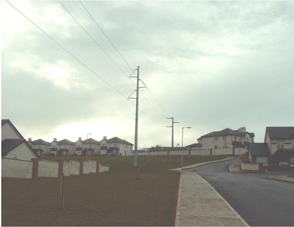
Figure 4.14: 110 kV Monopole Overhead Line in Cork
