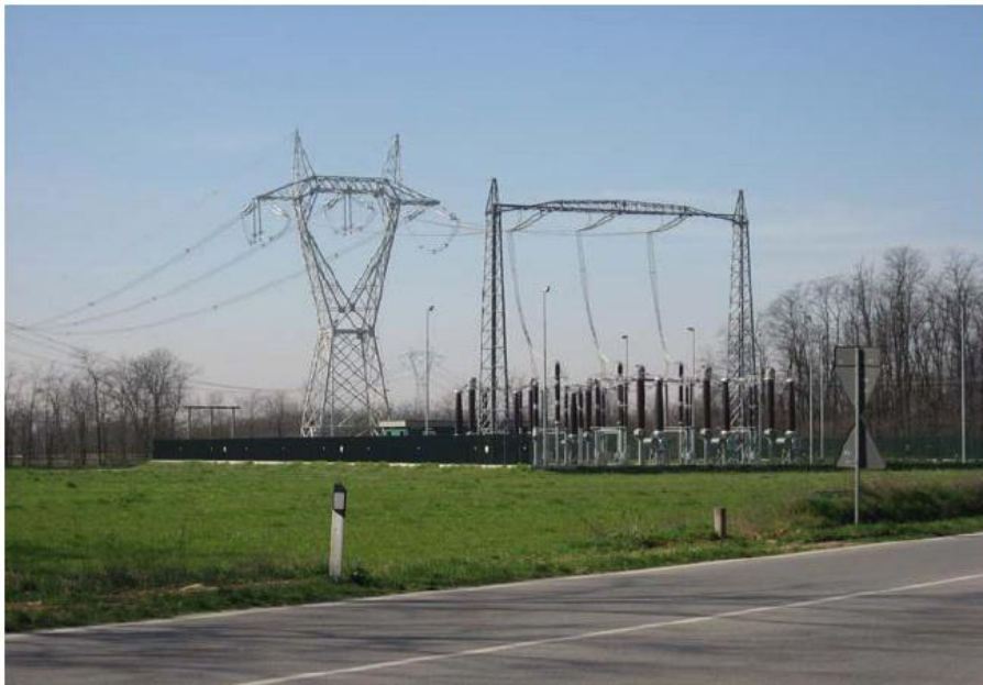
Figure 4.11: Example of a 400 kV Underground Cable to Overhead Line Transition Station
