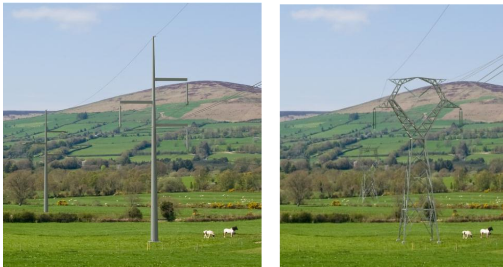
Figure 4.16: ‘Atkins’ Monopole Design and Proposed IVI Lattice Tower
